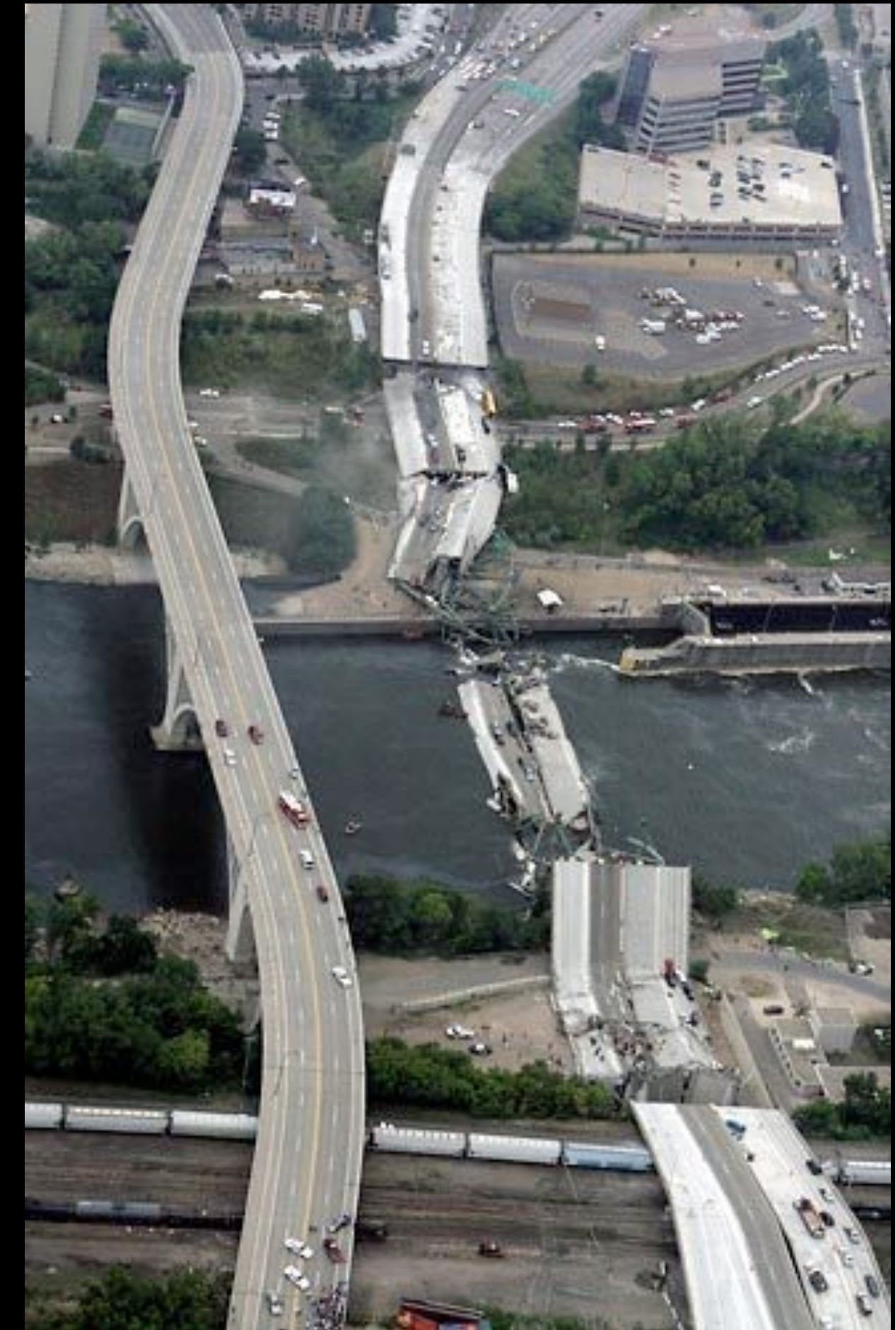
I-35 Minneapolis 2007 collapse
