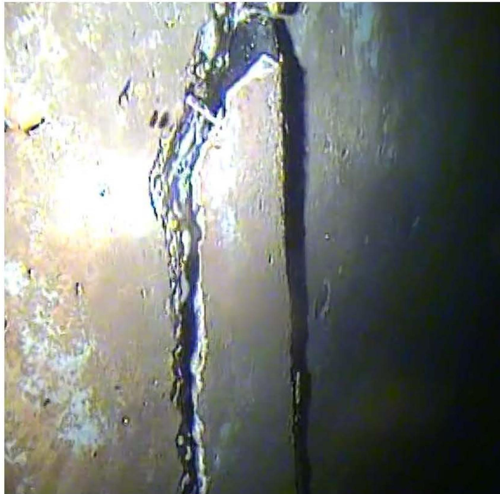
Photo # D1 – Wall spall at wall joint from diver's video (top portion)
